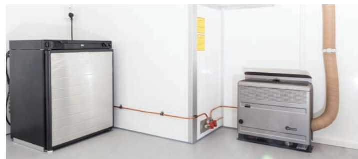
3-way refrigerator can be powered by gas, 12V or 220V electricity.
