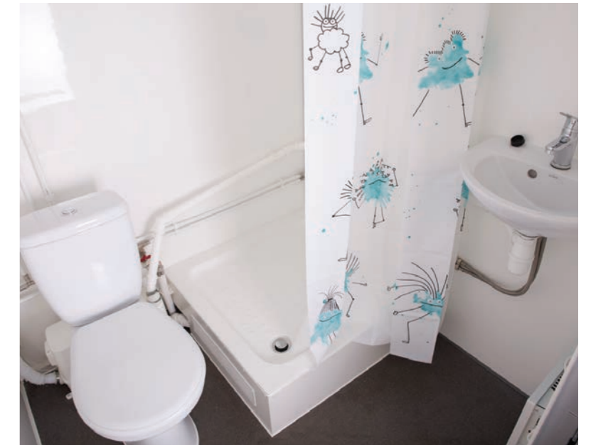
Ceramic toilet bowl, ceramic sink, shower, grinder and a boiler in the bathroom. Certified heater to withstand wet conditions.
